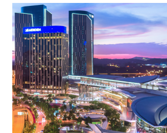
IOI City Mall Putrajaya, Malaysia
